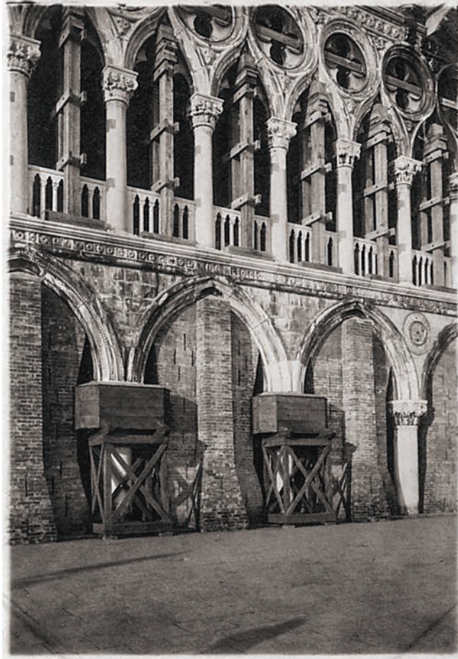
Figure 21: Doge's Palace reinforced to withstand bombing, Venice, ca. 1915. Photographer unknown.
